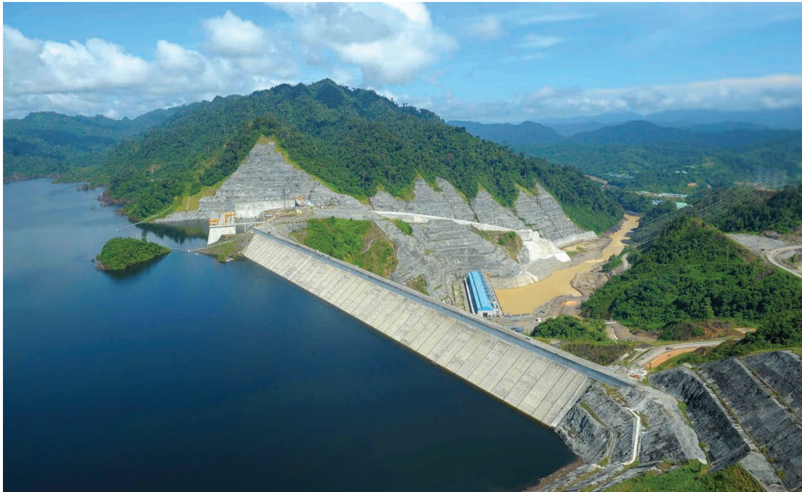
The Bakun hydroelectric project located in central Sarawak, Malaysia, features a 205m-high concrete-faced rockfill dam
